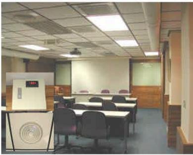
The push-pull ventilation system was adopted for controlling the flow path, and a pressure difference sensor was installed in the room for deciding to push or pull. Moreover, the ultraviolet disinfect instruments were installed at the intakes of the air conditioner to decrease the concentration of microbes.
